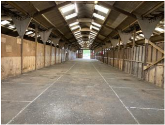
Photo shows example of one bay within Cattle Sheds
